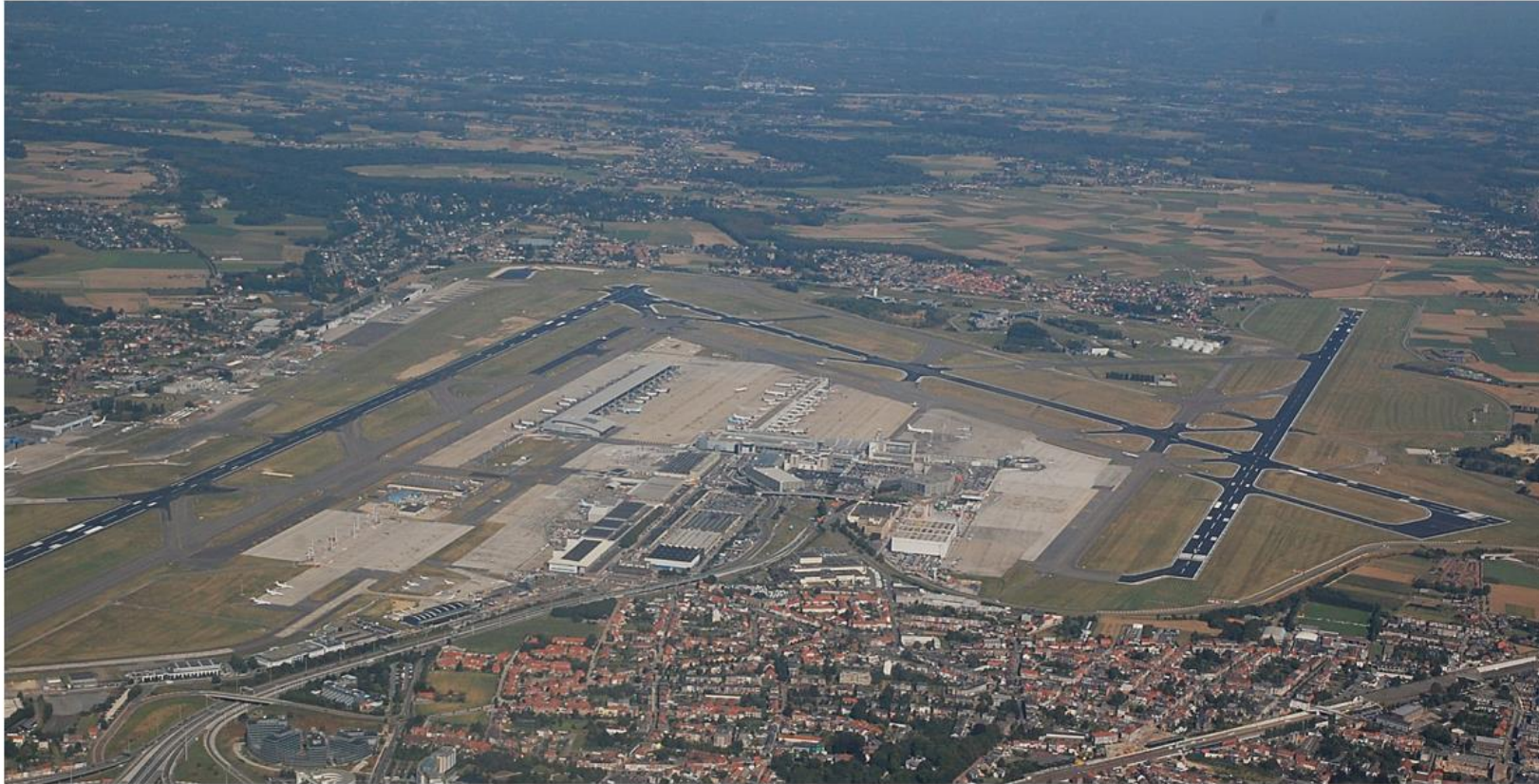
FIGURE 6.1 The area occupied by high-capacity modern airports, such as the Brussels Airport, may reach tens of squared kilometers and requires extensive terrain leveling.
